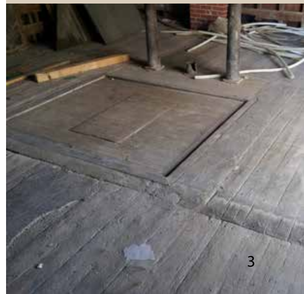
A scale built into the floor was used to weigh outbound freight.
