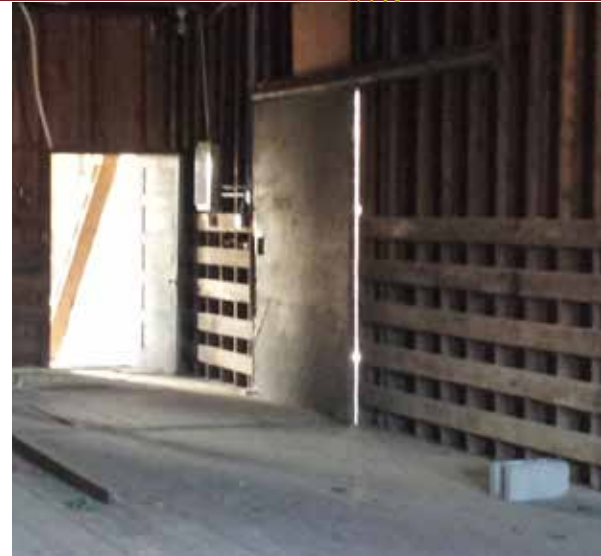
The warehouse portion of the freight station had unfinished interior walls, with horizontal boards spaced along the lower portion of the walls. They protected the walls and were useful when stacking and securing freight.
